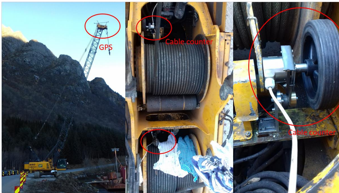
Figure 6 – location of cable counting sensors.
