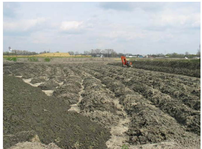
Treated dredged material is used to prepare a brownfield site for building. (Fasiver Project, Belgium).
