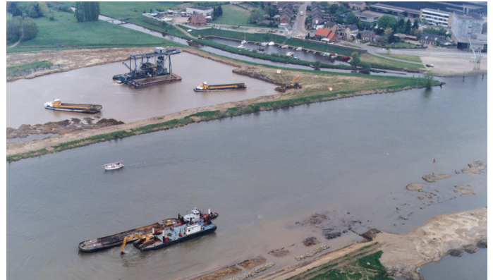
Figure 5. Dredging for flood management combined with sand and gravel mining in the river Meuse in the Netherlands
