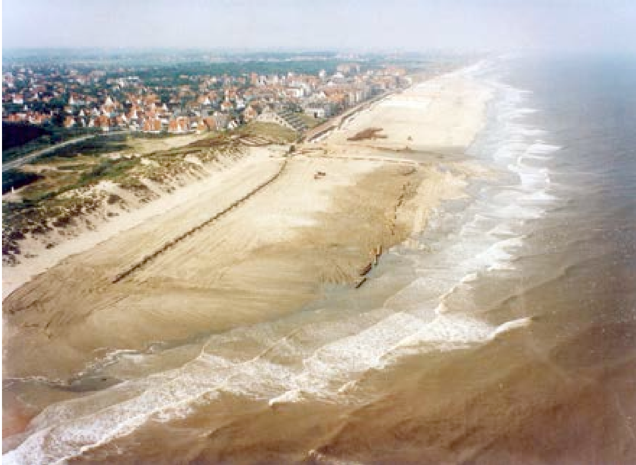
Profile Nourishment in combination by reclamation of the subtidal (submerged) beach at De Haan Belgium for sustainable and integrated coastal defence
